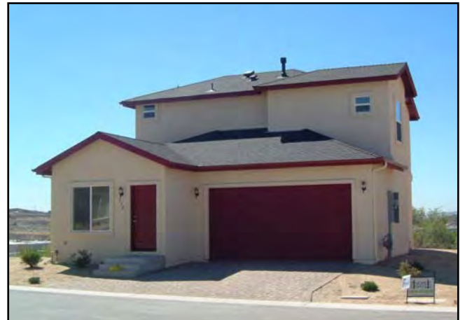
Highland Vista - Single-family housing
