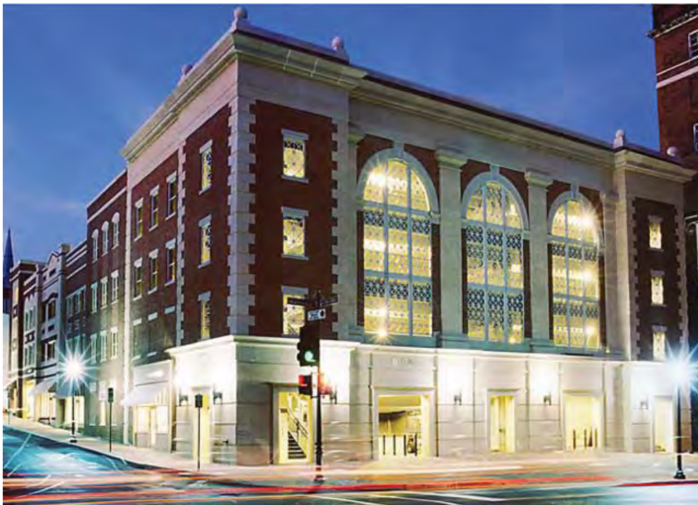
(Above) This Virginia parking garage incorporates architectural features of surrounding structures and provides commercial uses on the ground floor
